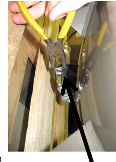
clean out cap Remove drain
