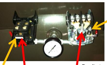
To adjust high pressure limit switch only adjust brass screw
